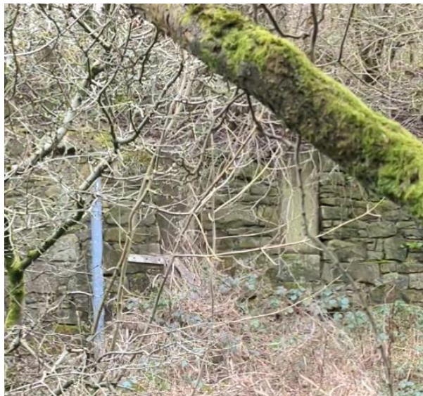
North side abutment
